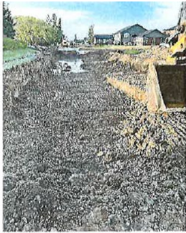
Over excavation of poor-quality material
